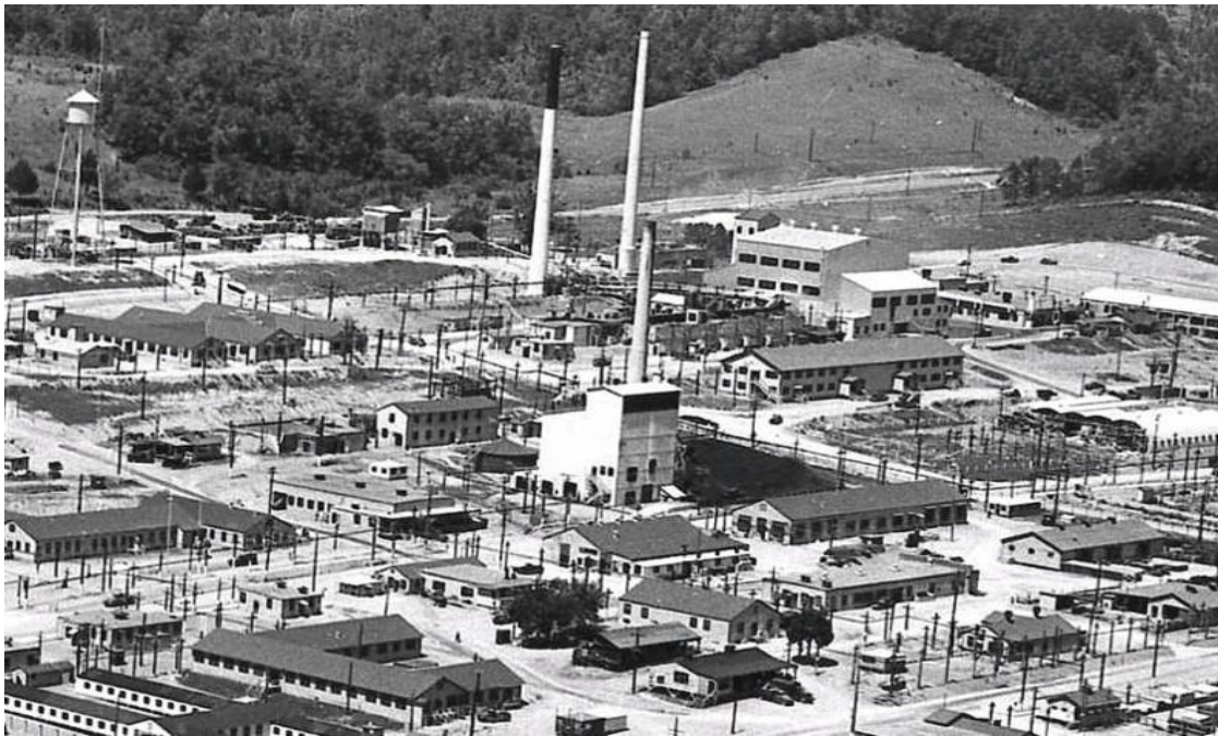
Oak Ridge National Laboratory's Graphite Reactor
